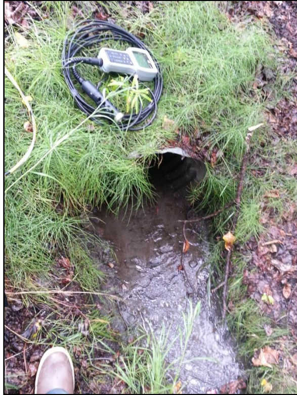
Photograph 9. Outfall SWM09 (499-1), Anchorage Football Stadium & Ben Boeke Ice Arena.
