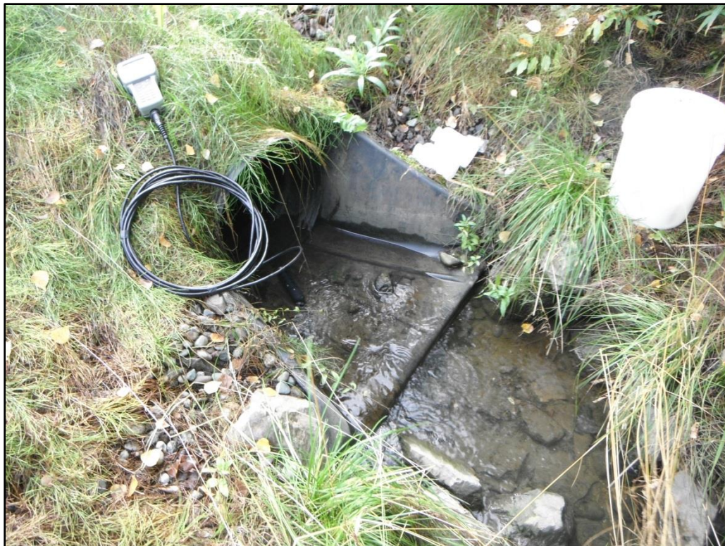
Photograph 4. Outfall SWM04 (1224-2), Fairweather Loop off Sylvan Drive.
