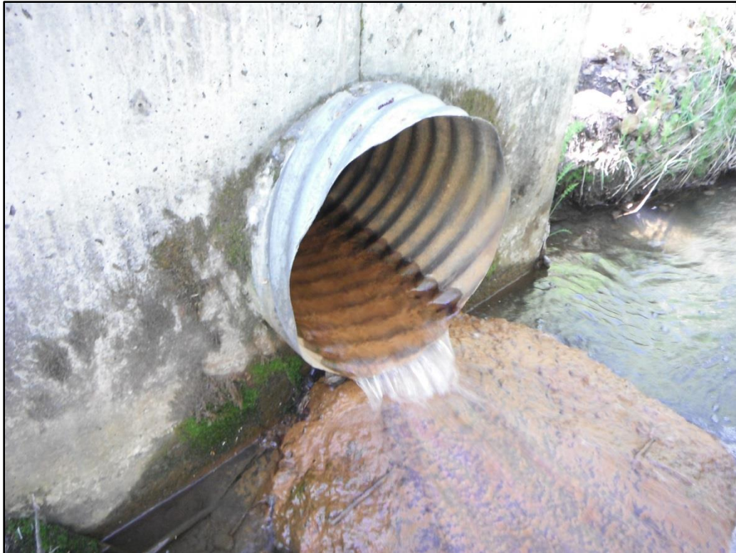
Photograph 10. Outfall SWM10 (525-2), Eagle Street at Chester Creek.
