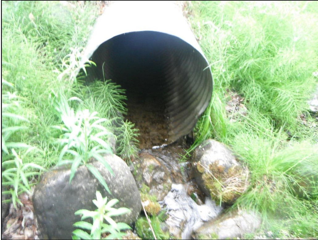
Photograph 3. Outfall SWM03 (1224-1), Fairweather Loop off Sylvan Drive.
