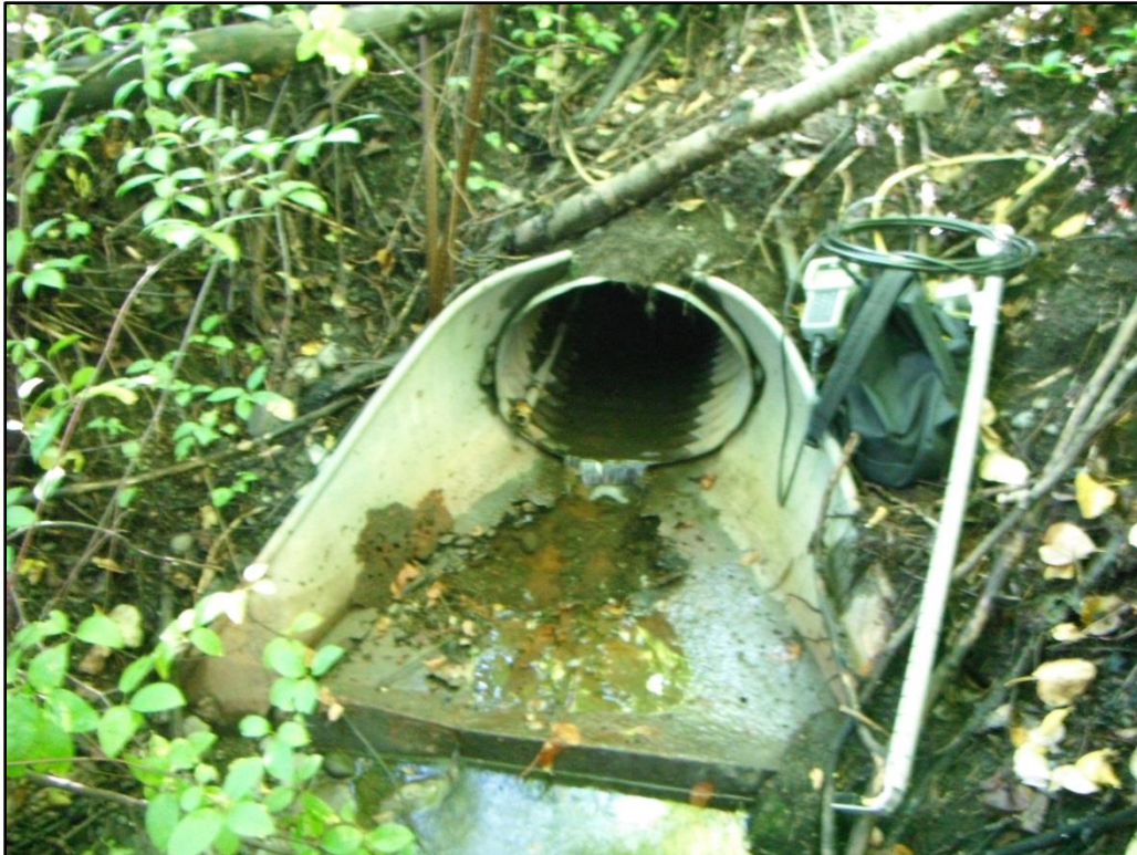
Photograph 6. Outfall SWM06 (314-22), Maplewood Street off of Northern Lights Boulevard.
