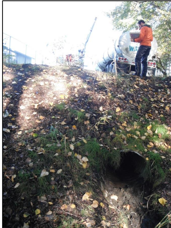
Photograph 12. Storm Drain Cleaning, Station SWM09, Storm #4.
