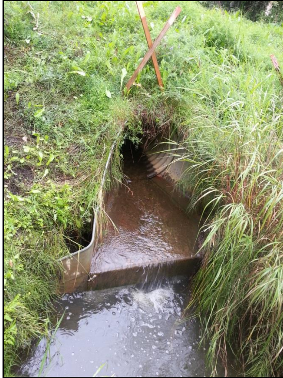
Photograph 5. Outfall SWM05 (207-1), East 56 th Avenue at Save School.
